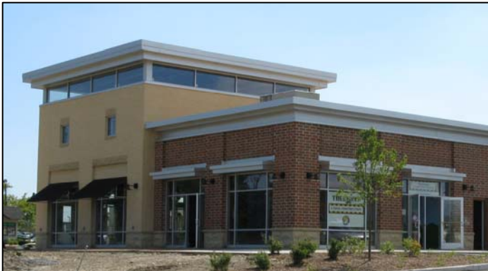
Smiling Georgie Porgie's used the CDBG-RLF proceeds to construct and renovate their new location to expand into another sector of the market.
